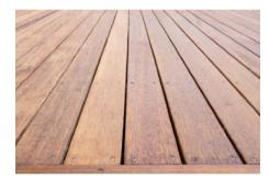
Merbau is a hardwood from Northern Queensland and South East Asia with a rich red colour. It's a very common timber for outdoor use and is very hard wearing. We enjoy working with this timber because it's easy to work and holds fasteners well. Merbau is a tannin-rich timber which can bleed onto and stain surrounding surfaces.
