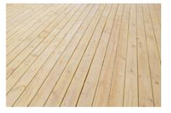
Treated Pine is often used for the structural elements of a deck. It is also a good lower cost alternative to hardwood decking boards. Because of its light natural colour it can be stained to a variety of colours. It's weather and termite resistant and is available in set lengths.
